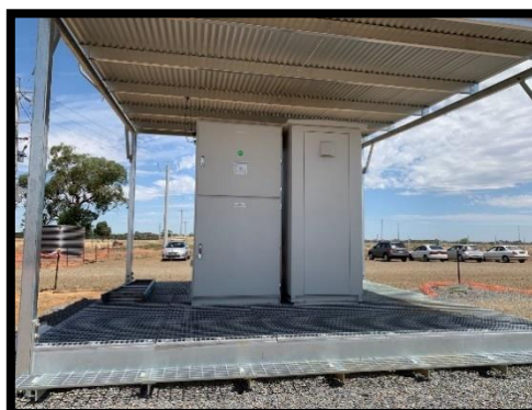
Figure 15 Typical HV switchboard and platform (Source: AC Energy)
